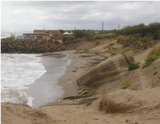
Erosion vs protection © CAHM
