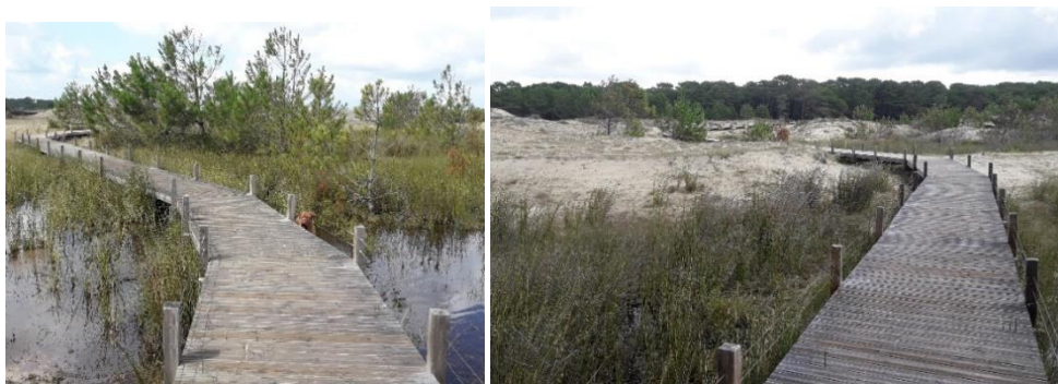
Figure 7: Platelage mis en place en 2018, (ONF, 2021)
