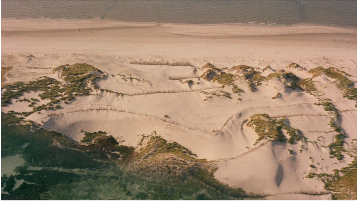
Figure 58. Rolling foredune at the Zandloper, North-Holland, October 15, 1990. A large number of notches have been dug on the foredune in a south-westerly direction. At the top and back (middle and bottom of the photo) the sand fences are visible that capture the sand in a controlled manner to guarantee a closed row of dunes. (Photo: Rijkswaterstaat)
